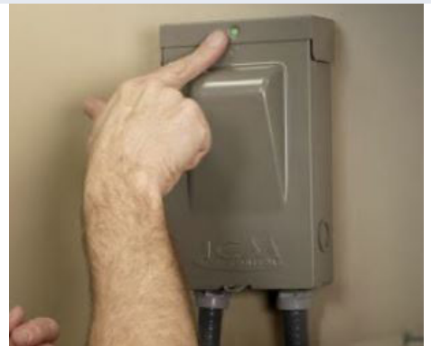
Figure 2: Integrated electrical disconnect with surge protector
