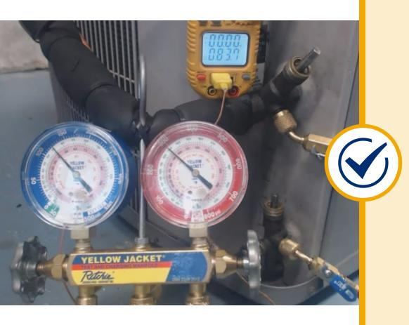
Always perform a leak test before loading the system with refrigerant
