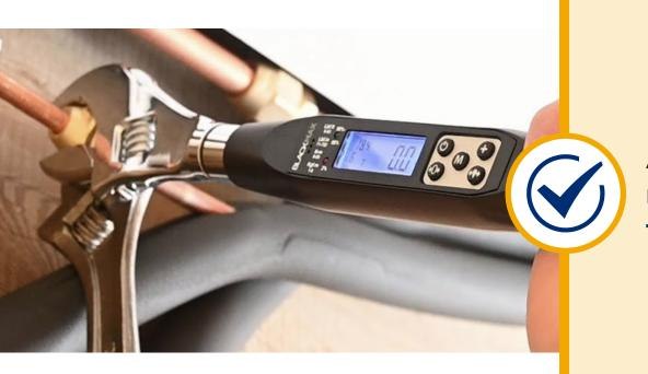
Always tighten flare nut to manufacturer specifications with a torque wrench
