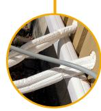
Step 11: Cover and seal the section to protect from moisture infiltration.
